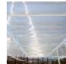
Tensile Structures Made of Metal
